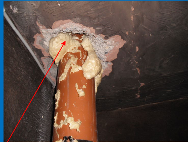
Improper sealing
