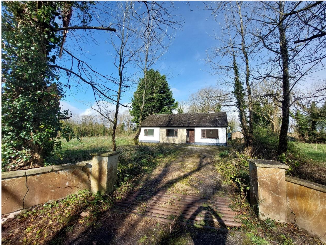
Figure 1.0 Front view of the existing dwelling (photo taken 27/03/2024)
