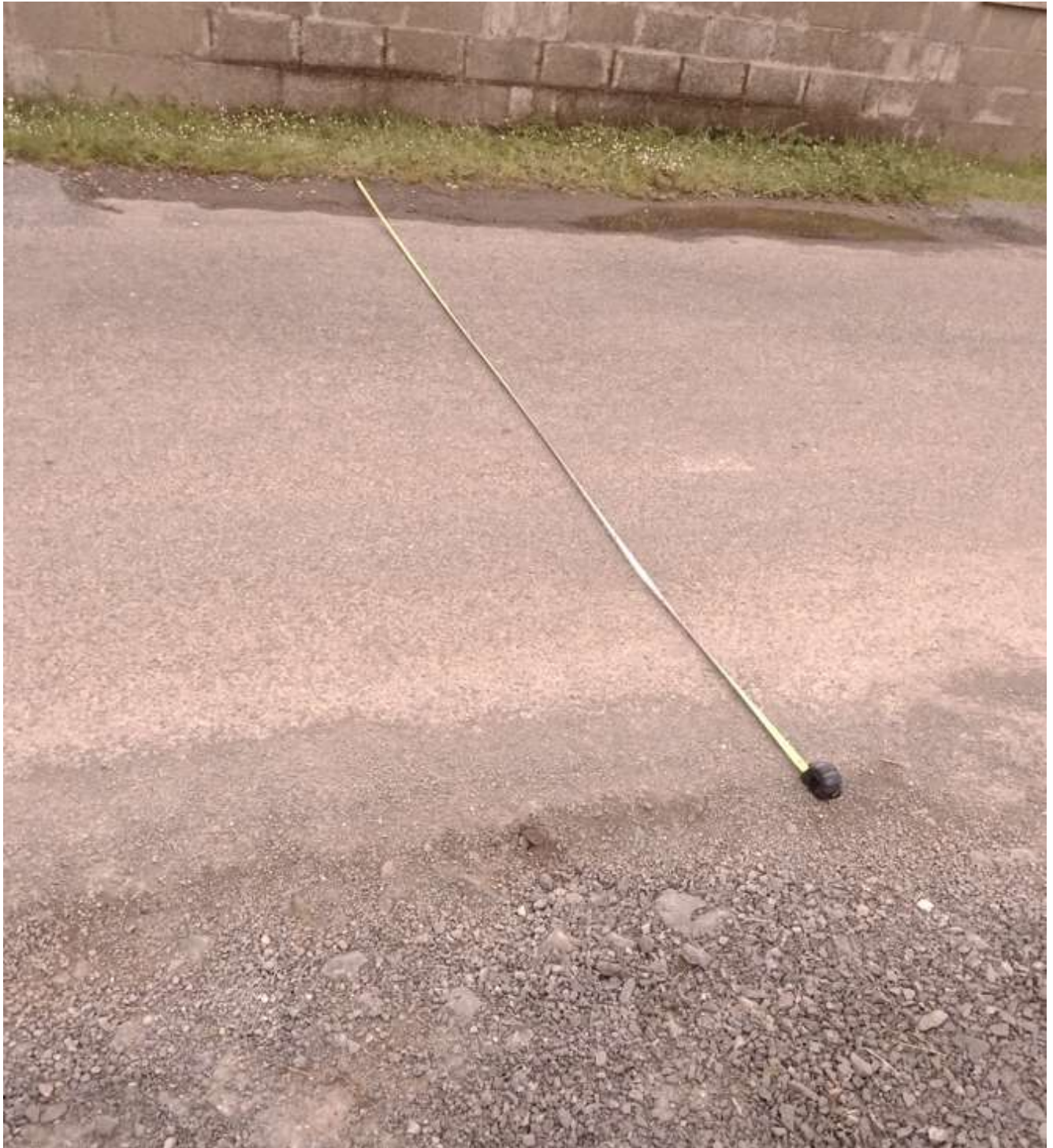
Width of road at 4.1 metres
