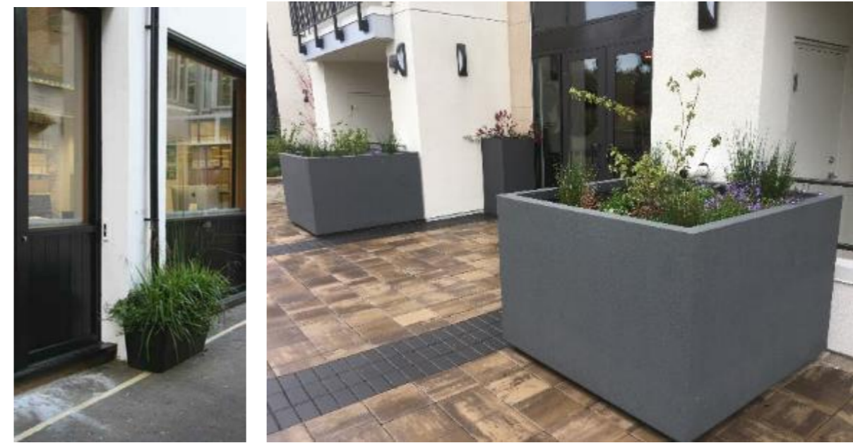
Figure 6-6 SuDS Feature to Capture Roof Run-off from Building Down Pipes
