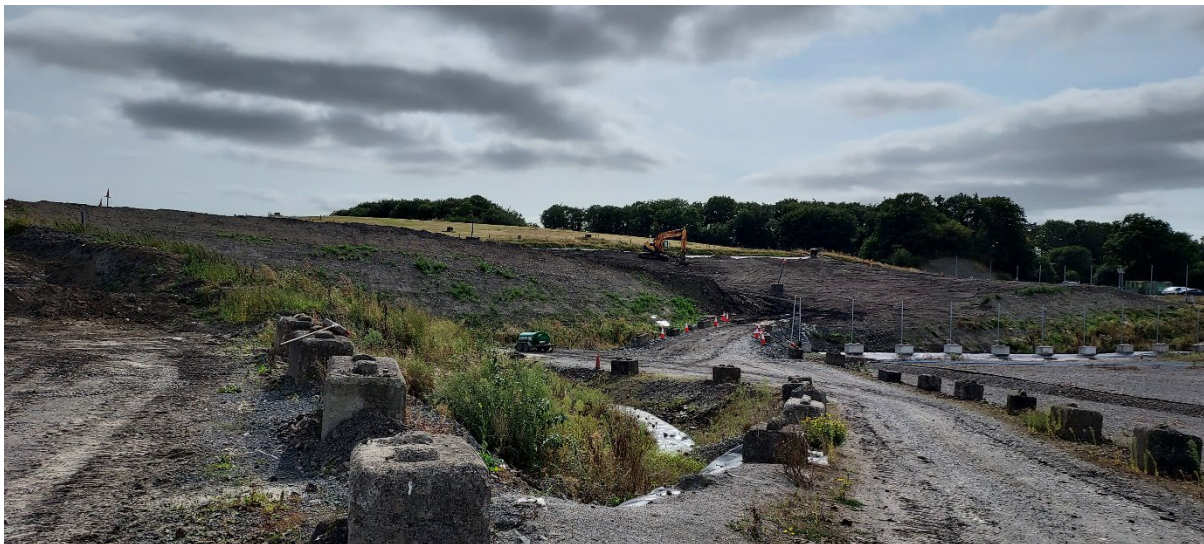
Ballaghveny landfill - view from the top of the ramp down to the waste tipping face in Cell 10B
