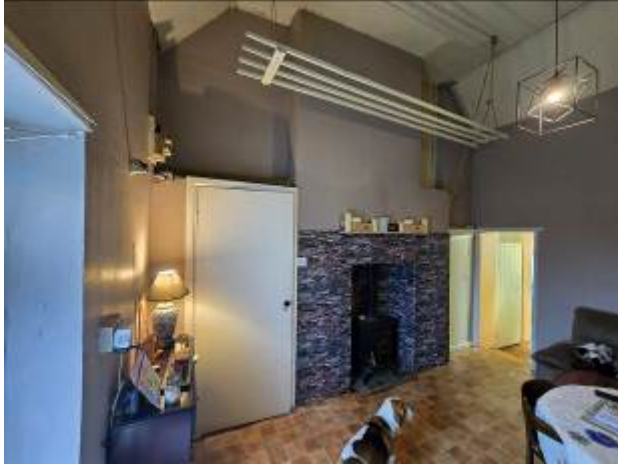
14.15.. Existing Central Dining Room. Soft Board ceiling to be replaced. Door way at rear to extension will become full height window.
