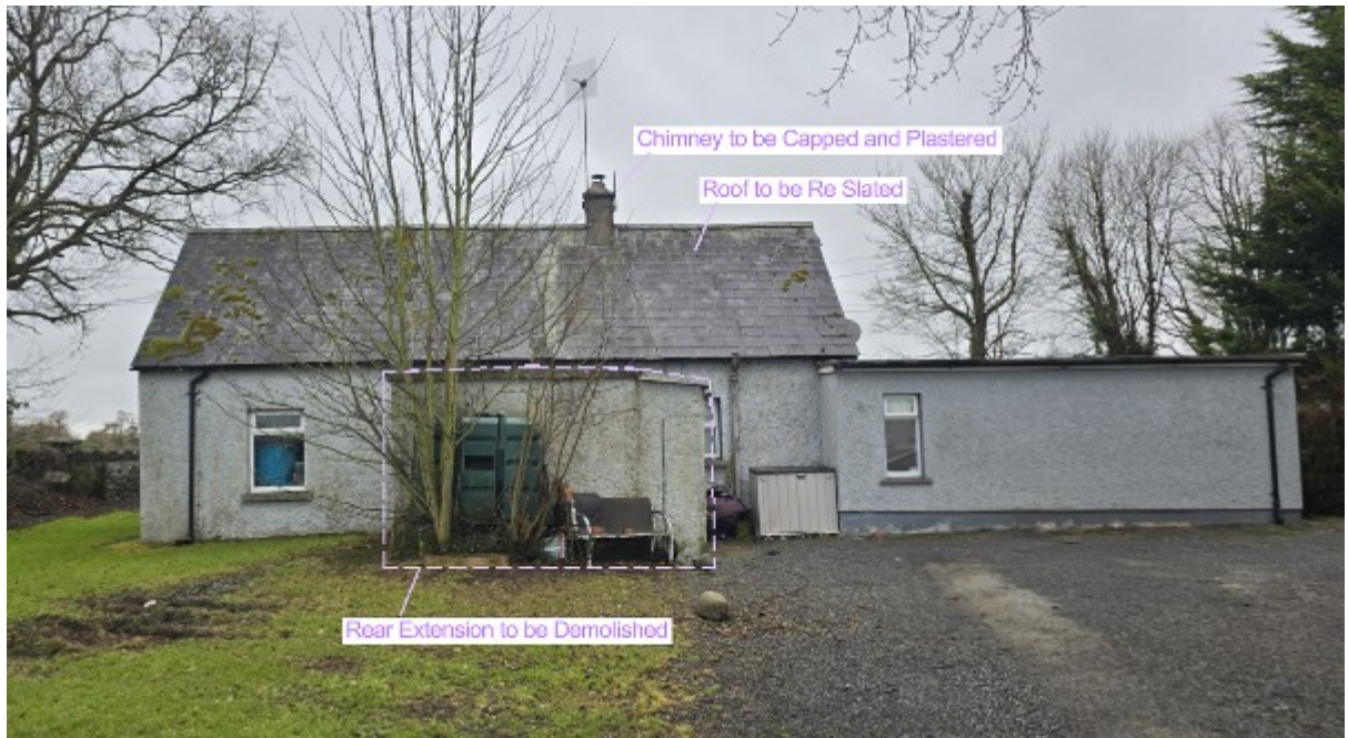
9. Rear Elevation, Alterations Highlighted
