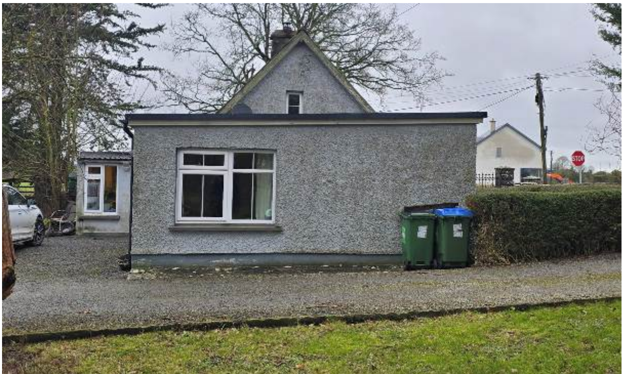
7. Side Elevation, South. Flat Roof Side Extension.
