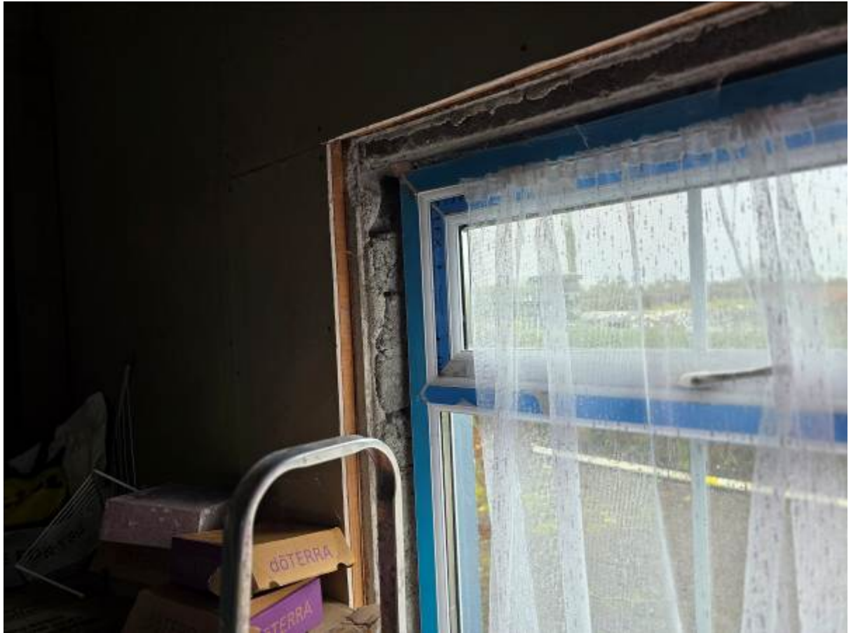
26. Dry lining on 215mm blockwork, form of construction of northern extension. Drylining to be replace in this room with Isover Optima system.
