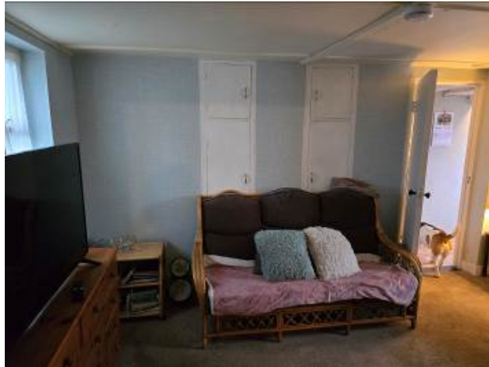
16. Existing Central Leving Room. Will become new Boot Room
