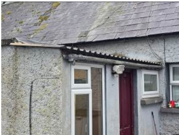
10. Rear Extension to be Demolished
